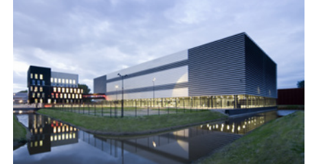
Equinix AM3 IBX data center exterior
